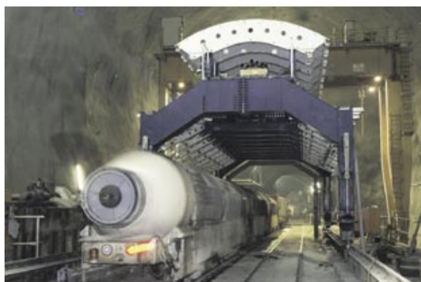
Montage Schalwagen Gotthard-Basistunnel, Oströhre.
